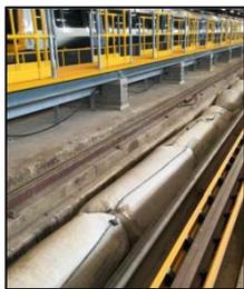
At Slade Green the Costain site team have identified a way to solve a problem with falls from height. They were working near to an inspection pit and use of temporary fencing was not viable. So the team came up with a novel solution to use inflatable air bags to fill the void in the pit while the works were being undertaken, the air bags could also be left in place at the end of each shift.
